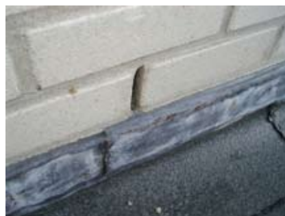
Controle waterdichtheid dakopstand.
