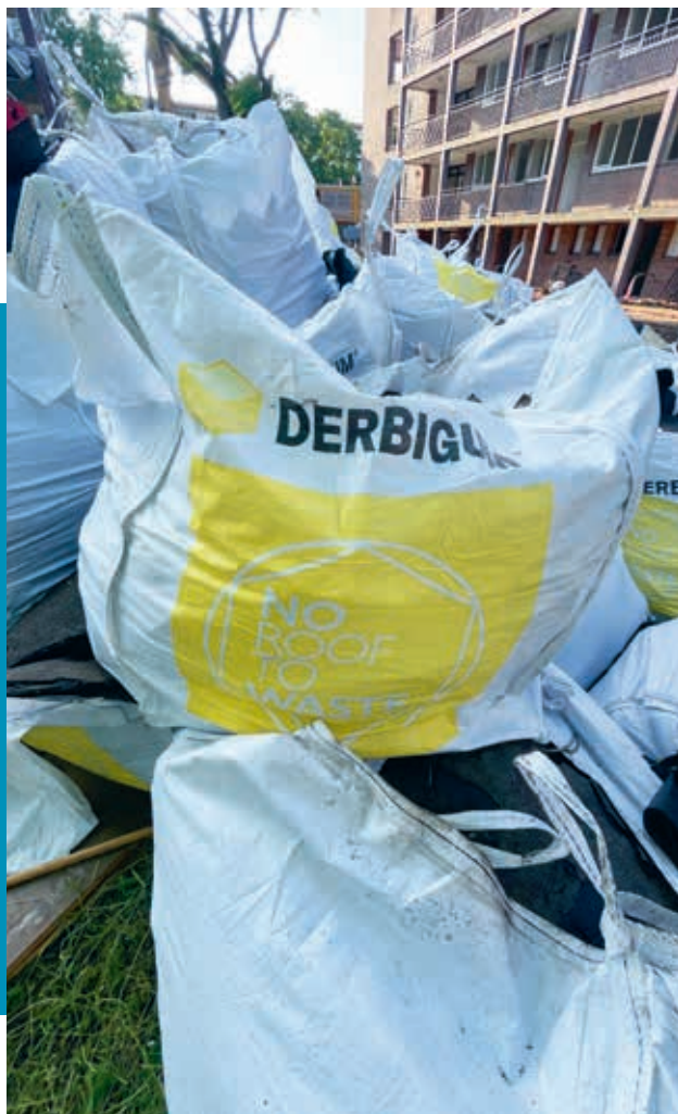
1.000 m 2 dakbedekking verdween in big bags.
